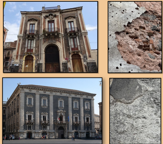
Examples of ghiara (upper photos) and azolo (lower photos) mortars in historical edifices of Catania city center.
